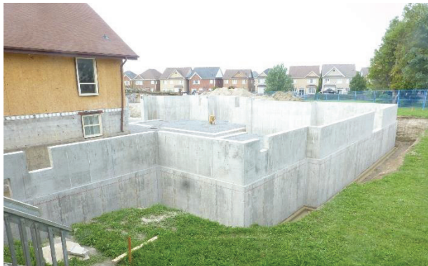
Basement walls completed
